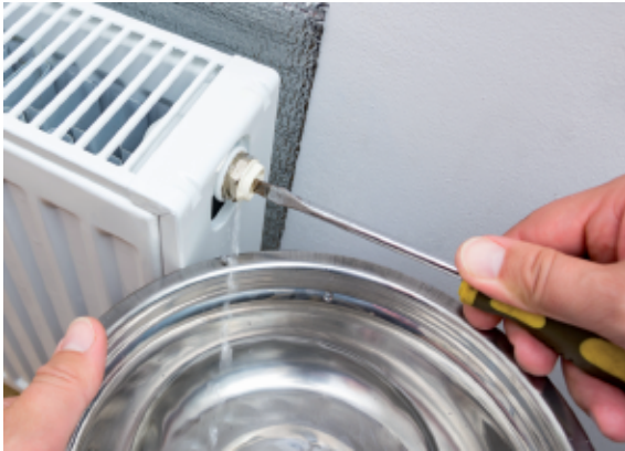
Bleeding with flathead screwdriver
